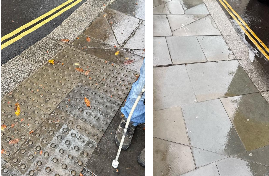
Image 5: Dropped curb with contrasted tactile paving, with no tactile cues on the steep slope on either side. Image 6: Dropped kerb with no tactile paving.
